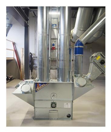
Elevator is easy to clean through large hatches. As an option, pre-cleaner A150 attached to top part keeps working area dust-free while conveying the grain.
