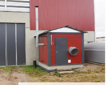
Heater room for overpressure heaters as option
