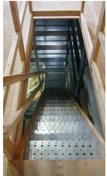
Sturdy stair steps and platforms
