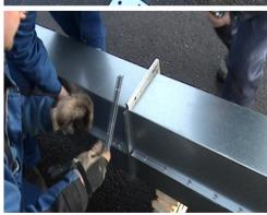
Fasten the rope to the end of the chain such that it can be pulled through the lifting tubes flaps ahead. By pulling the rope at the return side the chain is installed in the tube. To install the chain, pull the rope and at the same time help the chain to move into the elevator.
