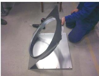
Connect the cover sheets with M8x16 and fasten the outlet collar (ILU 500/630) with self-tapping screws.
