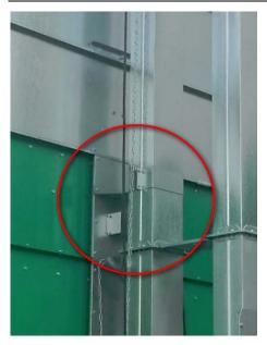
Check that the elevator is in a straight position (if necessary, check with an angle level and a spirit level). Tighten all connections carefully.
