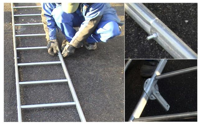
Attach the upper arcs to the ladder, the left is 5 cm shorter (1)923908, the right (2) 902000, by using the screws M8x35.
