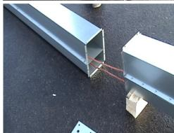
After that the tubes are connected to each other with L-brackets. Use hex screws M8x20.
