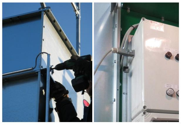
Connect the level guard cable to the electrical switchboard on the left side of the main electrical switchboard.
