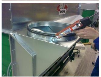
Place the cover sheet on the end plates, and fasten with M8x16. Use resin based mastic to seal the seams.
