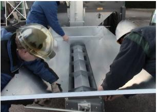
Connect the bottom sheets of the hopper to each other with screws M10x20, and fasten to the feeding auger with M8x16 (parts 1, 2 and 3). After that attach the intermediate supports (4), the reinforcements (6) and legs (9) on both sides of the hopper with hex screws M8x16 and M10x60.
