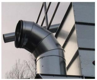
Place the elbow (BFU 500/630) on top of the channel aspirator, fasten with self-tapping screws.
