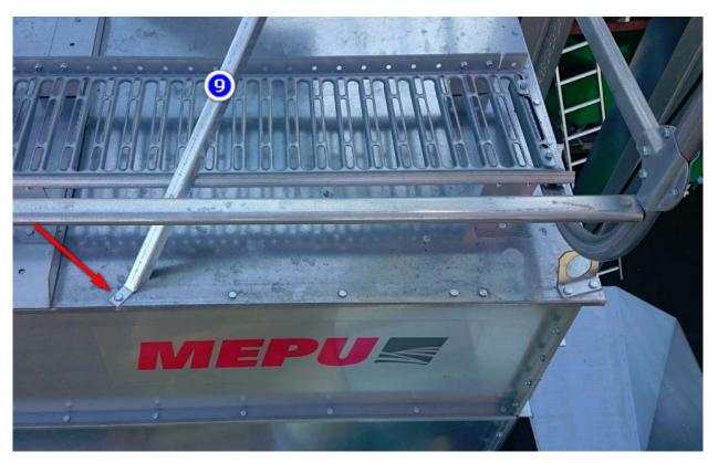
Elevator supports (lower) 2 pcs (part 9) are installed on both sides within the grain container, according to the image.
