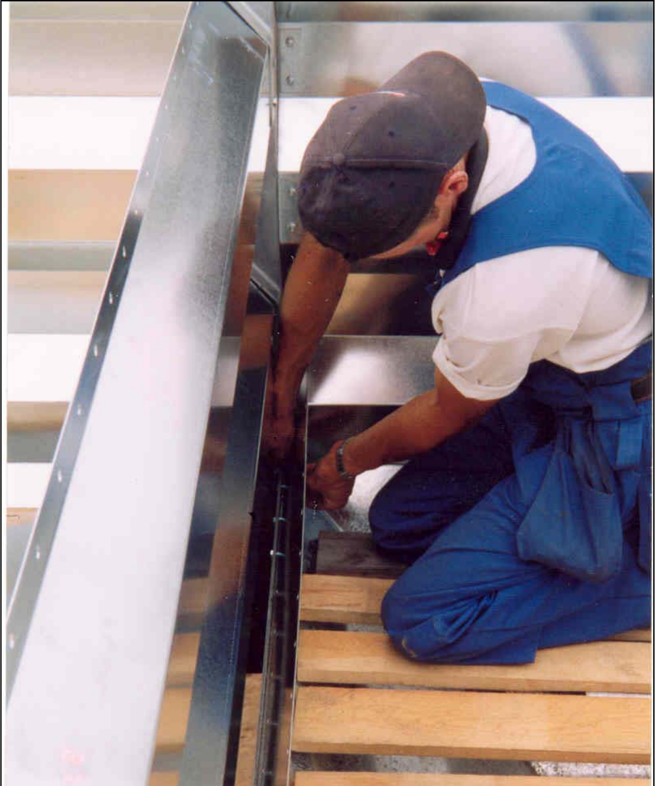
Installation of the silo cone spacer plates.
